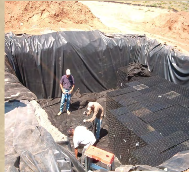
Construction of an Underground Structural Storage Tank in Rancho Viejo, New Mexico
