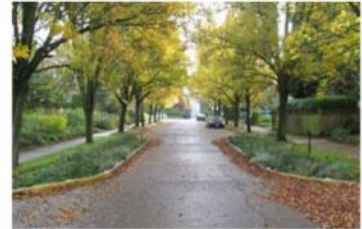
Stormwater infiltration planters along the street provide treatment and storage of street runoff. The infiltration planters narrow vehicular street widths to provide traffic calming and safer streets.
