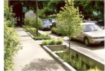
Curb openings allow stormwater to be conveyed from the street's gutter to stormwater infiltration planters.
