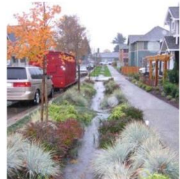
A stormwater infiltration garden located along this residential street treats runoff from the street and roofs of adjacent buildings.
