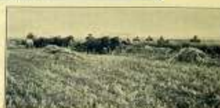
View of the Low Water Area, Irrigation Area, near Denver.
