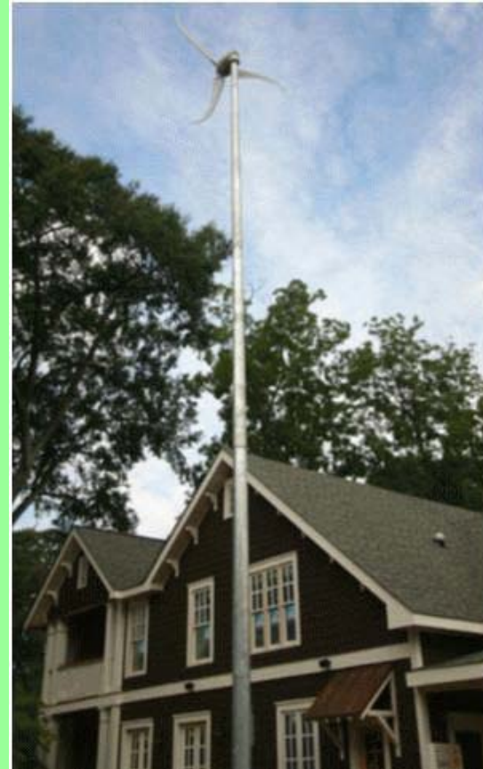
The installed 45 foot tall turbine
