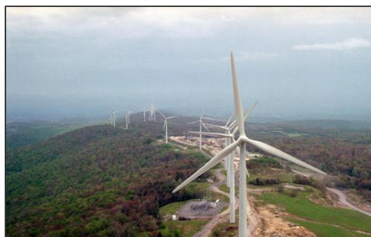
*According to NREL, the 44 turbines at the Mountaineer Wind Energy Center in West Virginia pictured above produce a maximum of 66 MW of electricity. Each turbine stands 228 feet above Backbone Mountain with rotor blades of 115 feet in diameter.*
