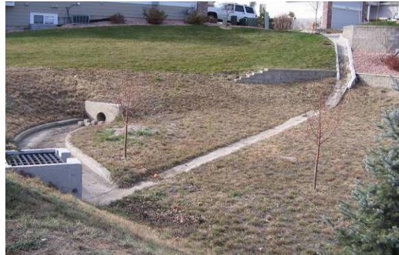
Connected impervious areas and trickle channels convey low flows and associated pollutants, which were previously absorbed, offsite directly to a waterway.
