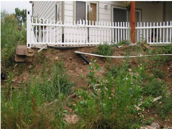
Example of waterway scour and destabilization from excess urban runoff.
