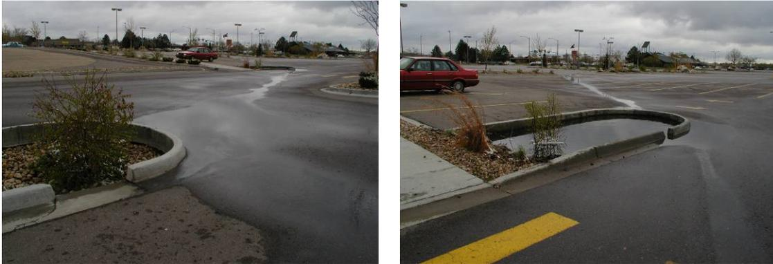
The PLD on the left should allow water to flow into it at the curb cut however the asphalt surface is not installed in a manner that allows water to flow through the curb cut. This causes the next PLD to receive excess flow.
