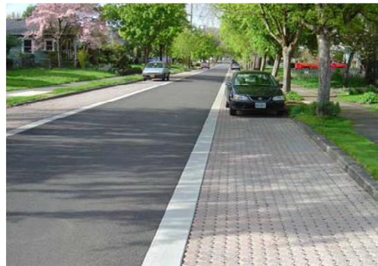
Runoff from a narrow driving lane can sheet flow onto a permeable paver system to reduce road runoff.
