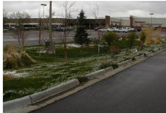
Multiple inlets may help reduce the erosion and sedimentation of a PLD.
