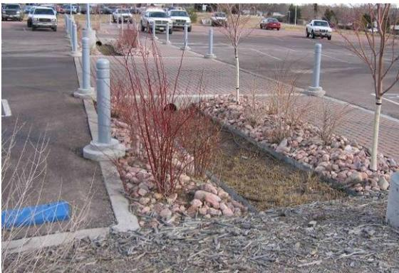
This parking area combines several LID elements: flush curbs with wheel stops, block pavers, porous gravel parking spaces and sumped landscaping to reduce runoff.
