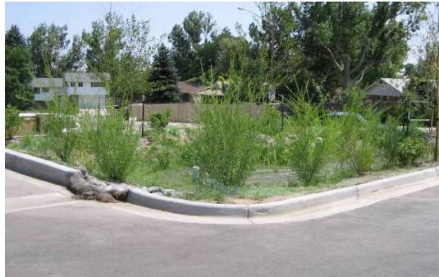
This PLD has a single valley pan inlet instead of multiple curb cuts. This property may benefit from more frequent sediment sweeping to reduce the sediment load that can flow into this structure.
